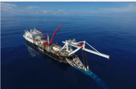
Gas Export Pipeline installation continuing
