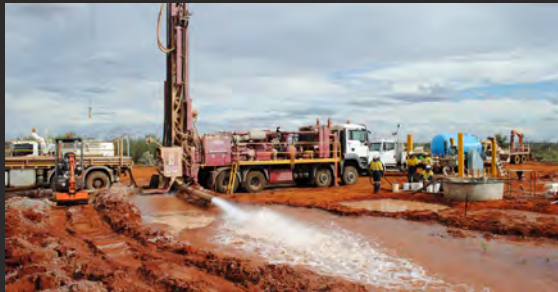
Water drilling at Nolans Site
