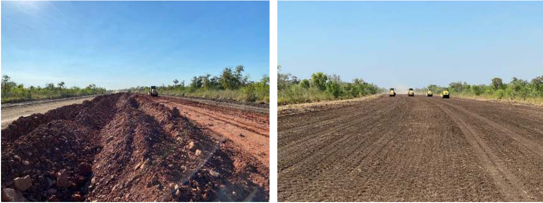
PHOTOS OF MOONAMANG ROAD CONSTRUCTION SUPPLIED BY MAIN ROADS WA
