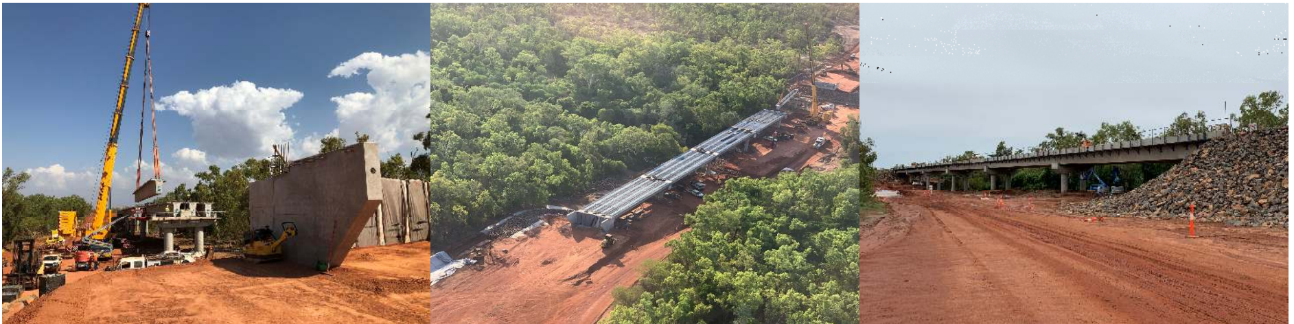
Keep River Bridge Construction
